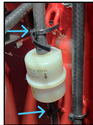
Figure 3 Zip Ties Securing Fuel Filter
