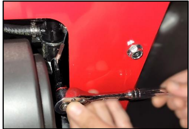
Figure 15 Removing Positive Wire from Fuel Transfer Switch
